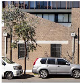
Splayed brick parapet
